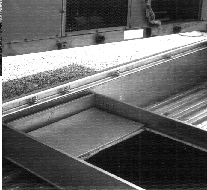
Inside view of CMAB showing cadmium plated 1"(25mm) deflection springs.
